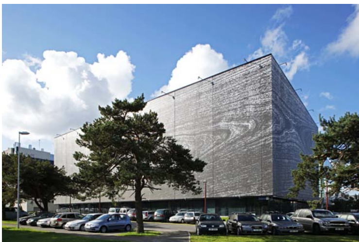
Facade covered by technical textile (Photo: Rait Agurajuja)
