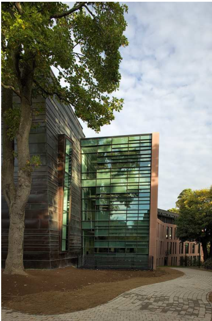
Facade Extension (Photo: Wilson Architecture)
