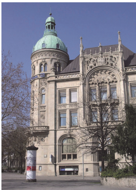
Fig. 1 'Deutsche Bank' building at Hannover, constructed with Obernkirchen sandstone.
