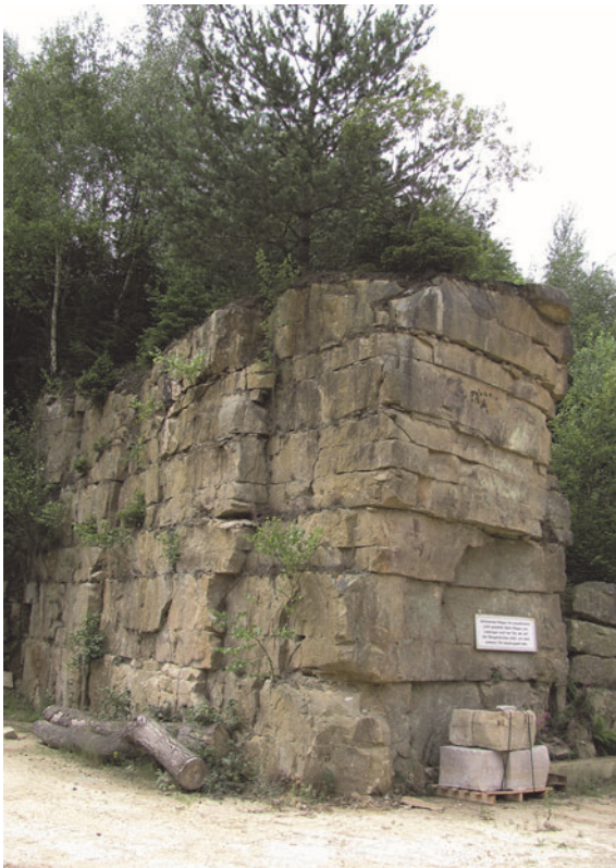
Fig. 2 Outcrop exposing almost the original quarrying height, as can be seen opposite to the sawing hall.
