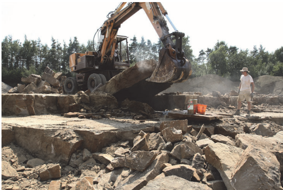
Fig. 7 The massive sandstone layers above the Lower Level trackway layer can only be removed with an excavator.
